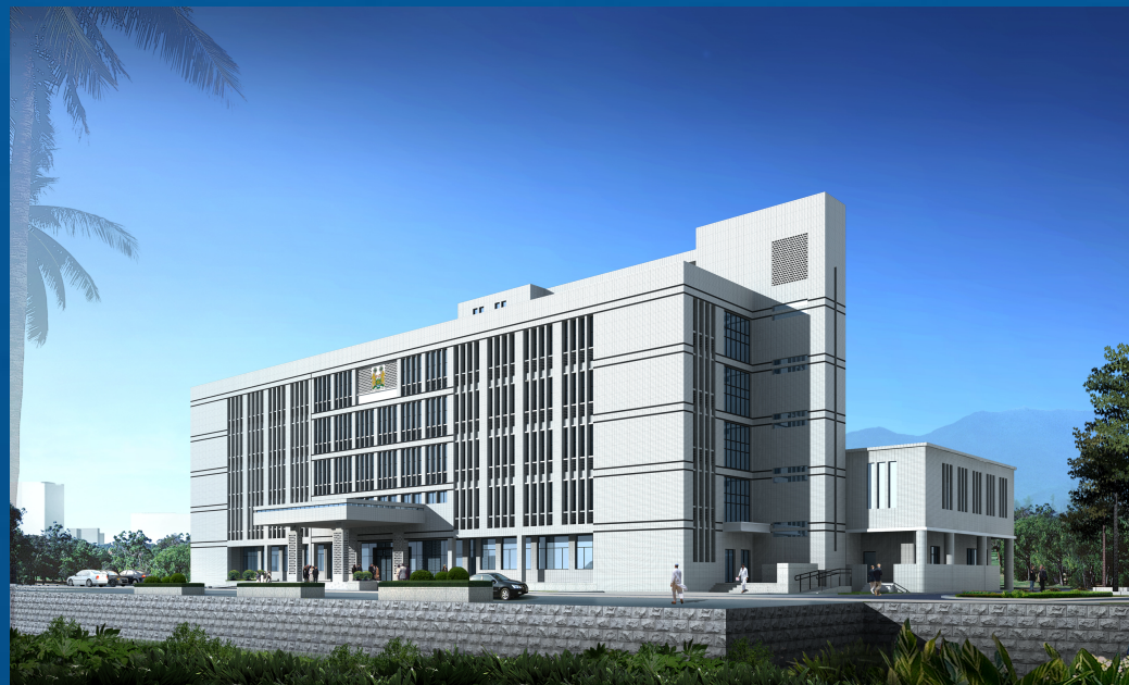
塞拉利昂外交部办公楼项目 The project of the Ministry of Foreign Affairs building in Sierra Leone
