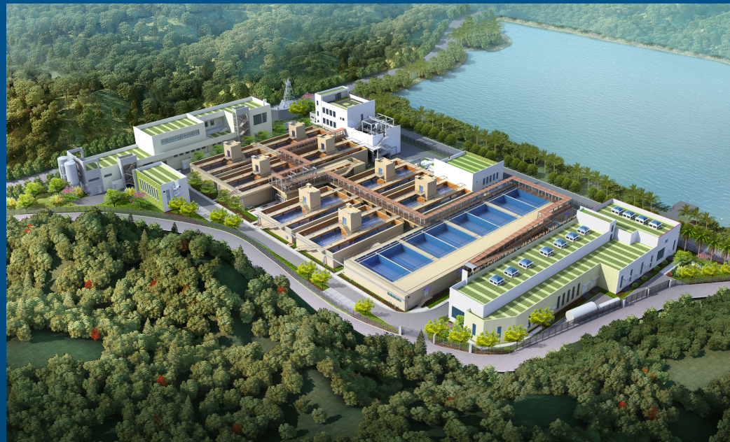
澳门石排湾净水厂项目 The San Pai Wan Water Treatment Plant Project in Macao
