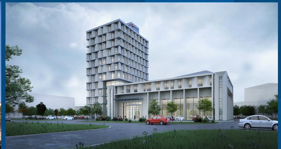
布隆迪国家税务局办公大楼项目 The project of the National Tax Bureau building of Burundi
